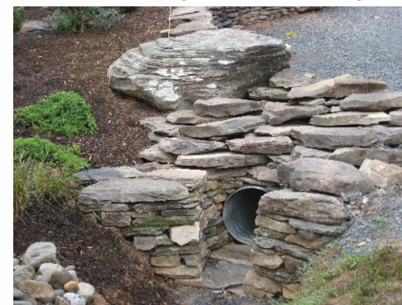
Retaining Wall Culvert Feature
