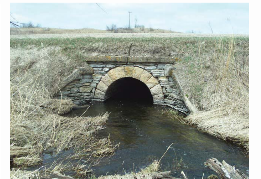
Stone Culvert Feature
